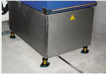
Small combined heat and power plant
